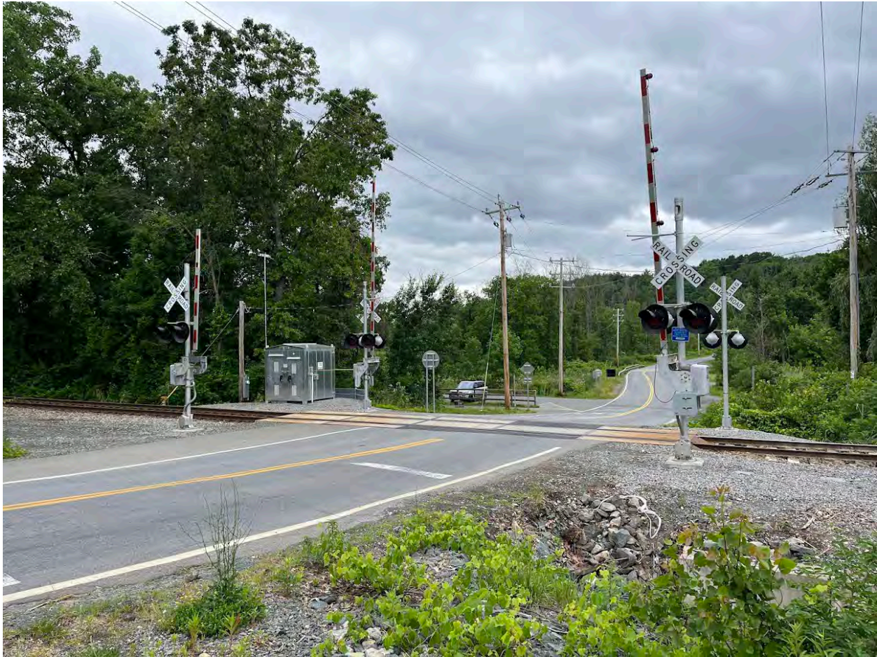
Photo of railroad infrastructure at the Zim Smith Trail parking area
