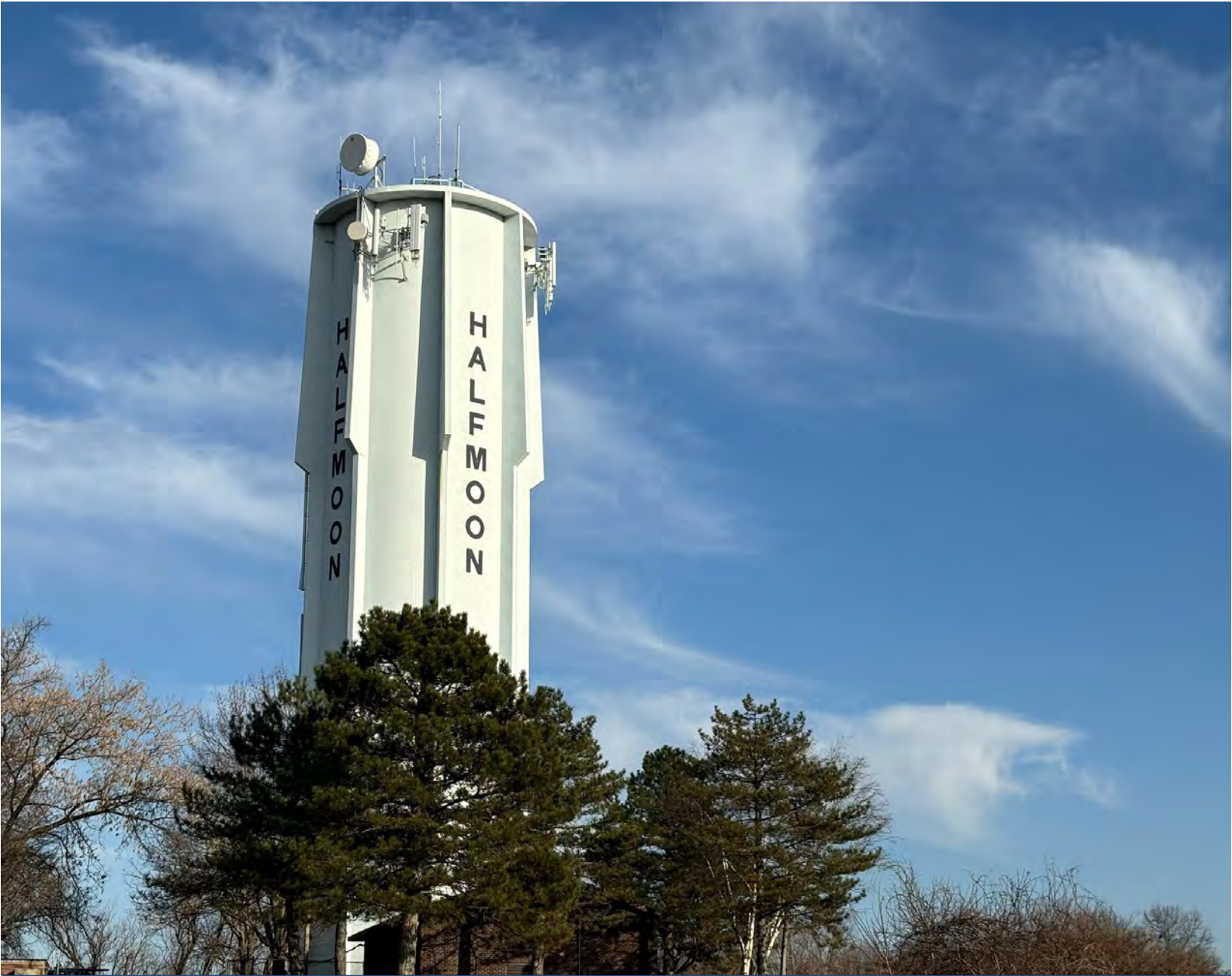
Photo of Water Storage Tank
