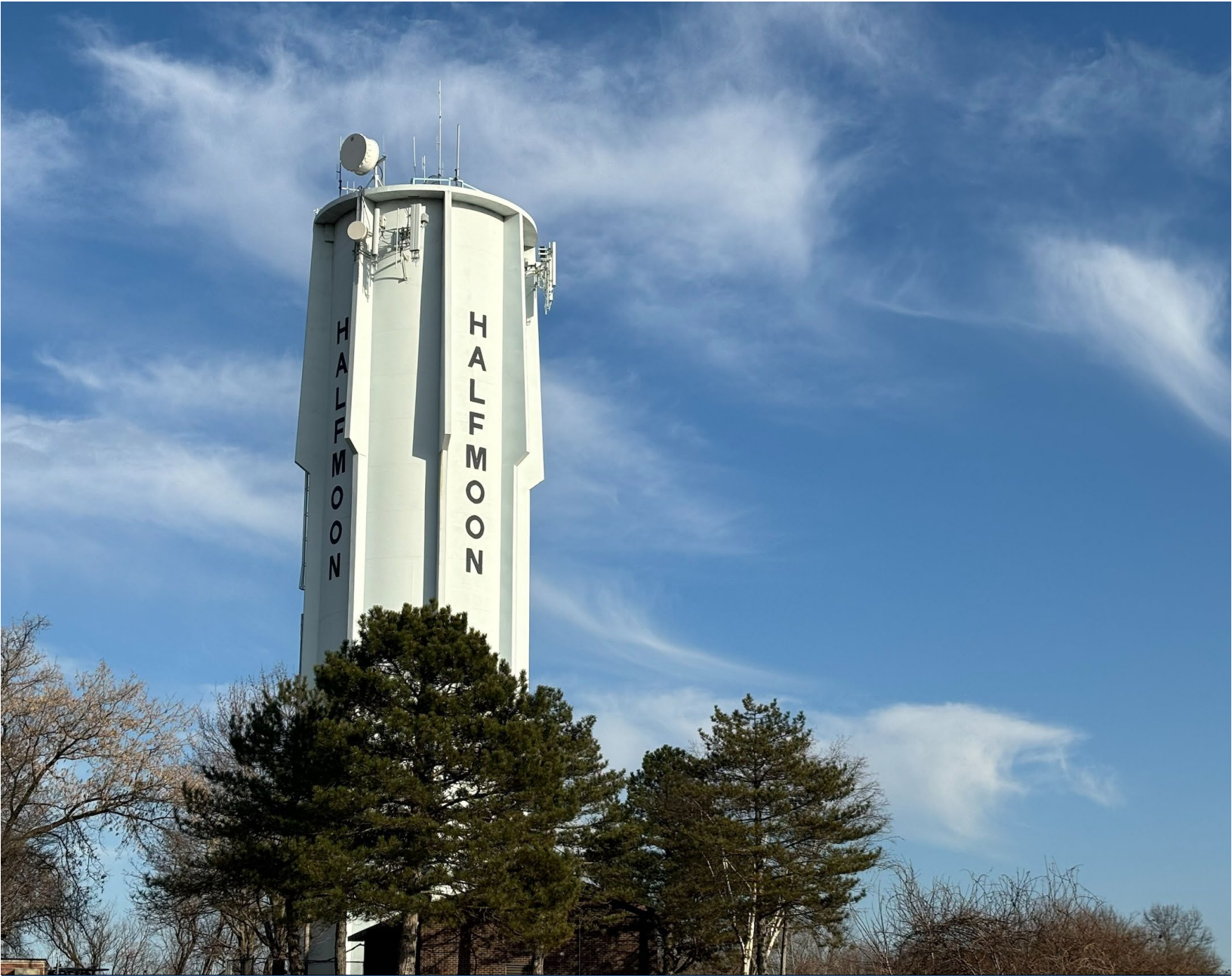
Photo of Water Storage Tank
