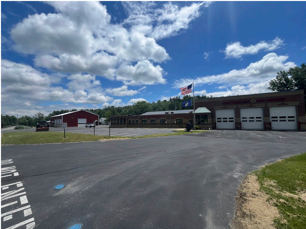
Photo of West Crescent Fire Department
