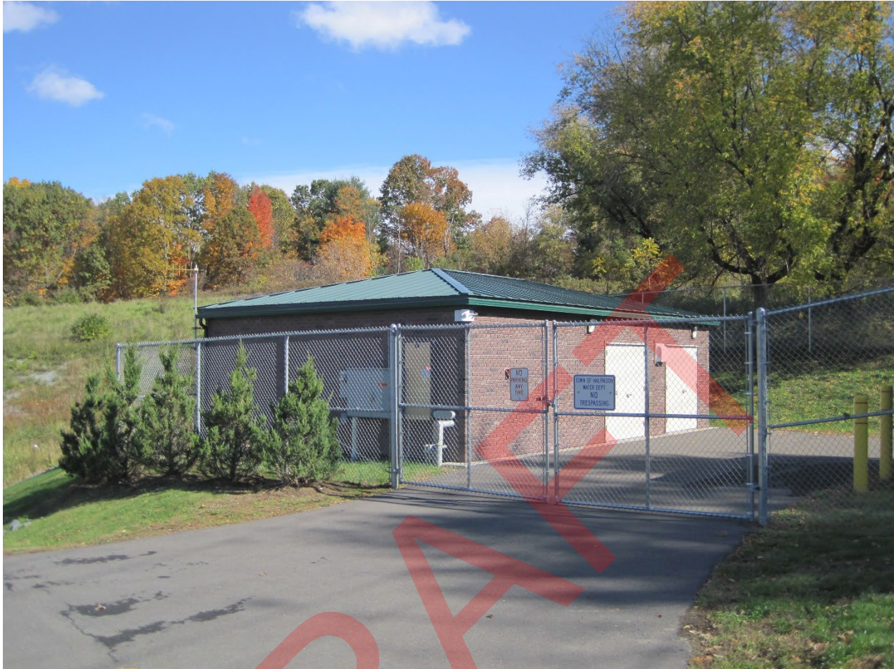
Photo of the Coons Crossing Road Pump Station
