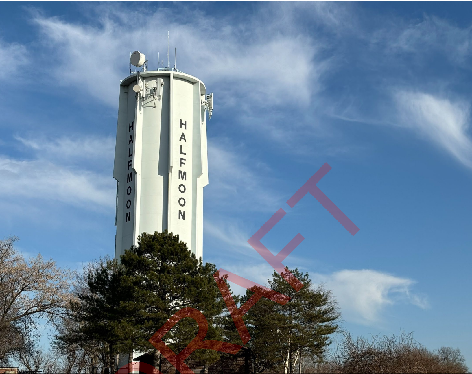
Photo of Water Storage Tank
