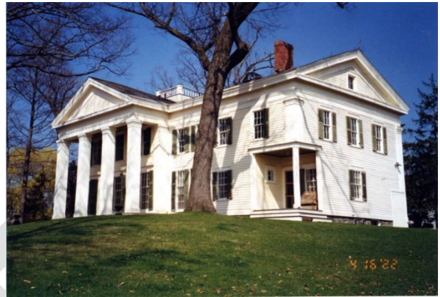
Figure X: The Oakcliff House from the rear or river view in the 21st century.
