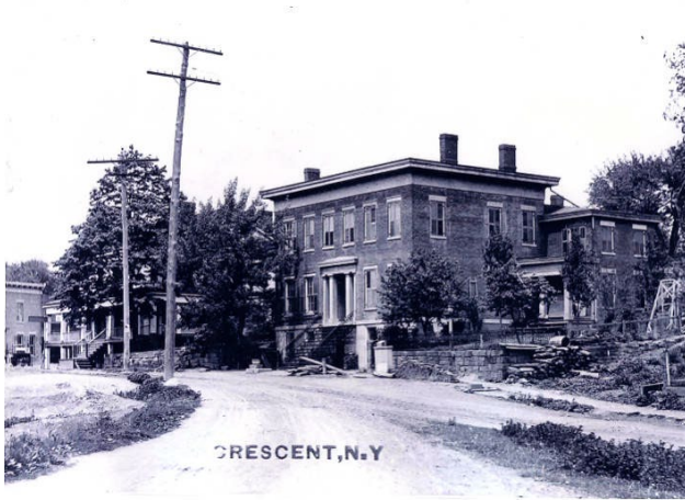
Figure X Noxon Bank Building looks northwest from Terminal Road. The image is stamped with "Crescent N.Y."
